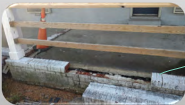
Damaged staircase
